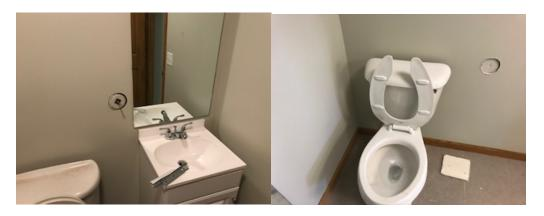
There was 1 toilet drain that was filled with concrete however the plumbing supply lines were still in place if it was ever to be turned back into a toilet area that drain line would need to be checked by a licensed plumber. This is a Consideration Item
