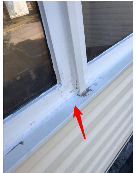
Caulk and paint on rotten windows
