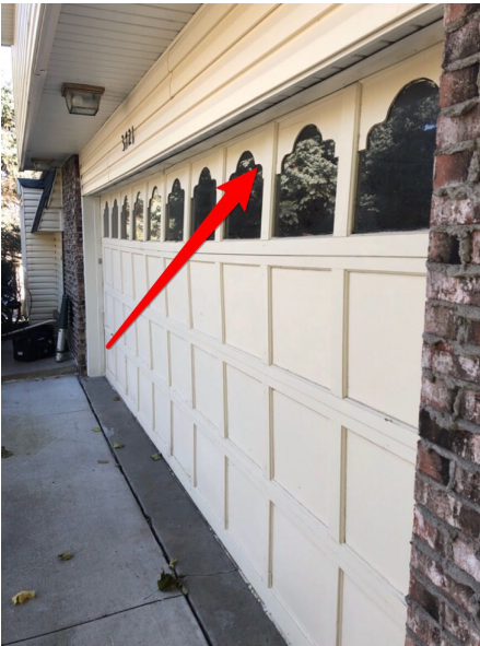
Door doesn't close and seal
