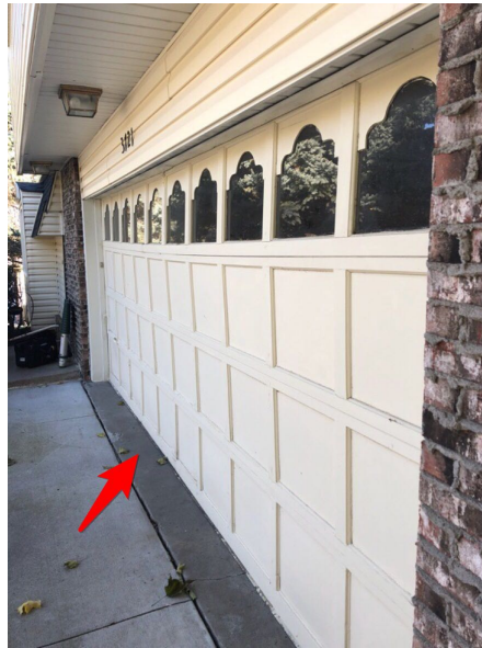
Rot near lower portions of door
